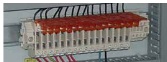
Primer uporabe varovalnih sponk / Application example of the fuse terminal blocks.
